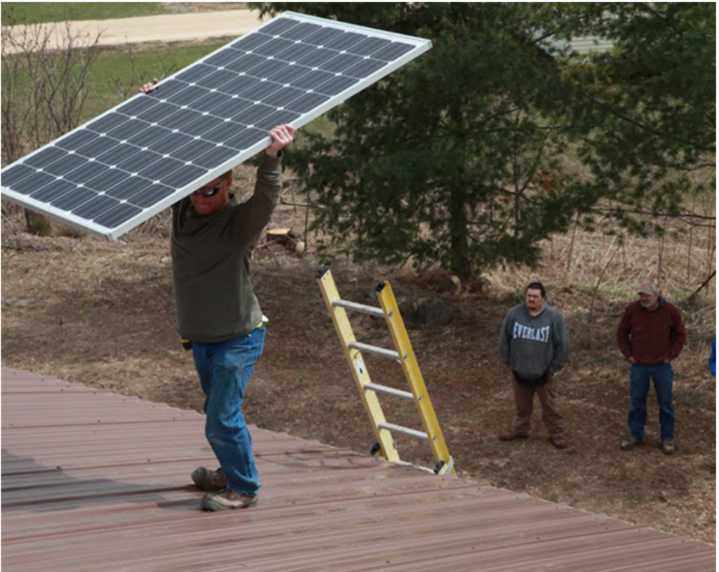
Installation of solar panel. Photo courtesy of D. Kakkak, CMN.
