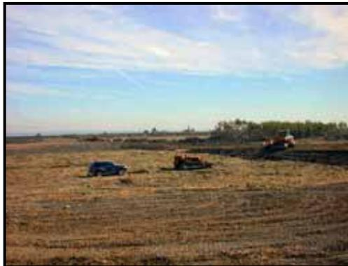
Dike construction material was originally to be obtained from within Cell 5, in the borrow area shown on the USACE drawings. This material was inappropriate, due to its water content and composition, therefore, material was conveyed from the offloading area to the cross dike location via 35-ton off-road articulated dump trucks.
