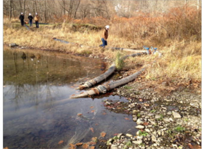
Figure 6-2. Self-supplied water acquisition site on a river in the SRB.
