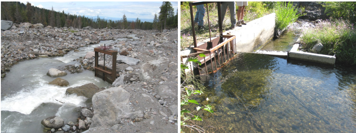
Figure D-4. Head gates used to control flows into a diversion (© 2014 Farmers Conservation Alliance, used with permission, http://farmersscreen.org/screen-projects/featured-projects/ ).
