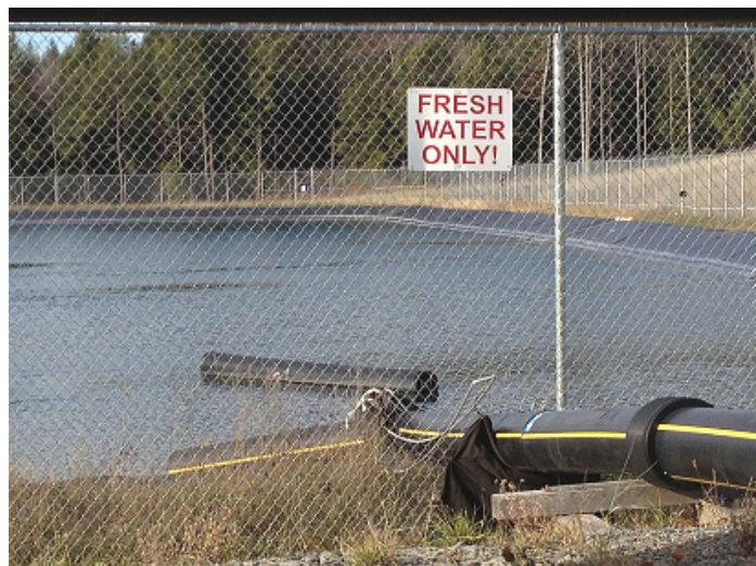
Figure 4-25. Photograph of O&G freshwater impoundment to service hydraulic fracturing water needs.
