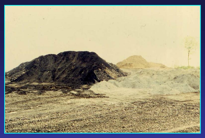
**Special Handling** – acidic or alkaline materials are identified, segregated, stockpiled, and selectively placed in the backfill.
