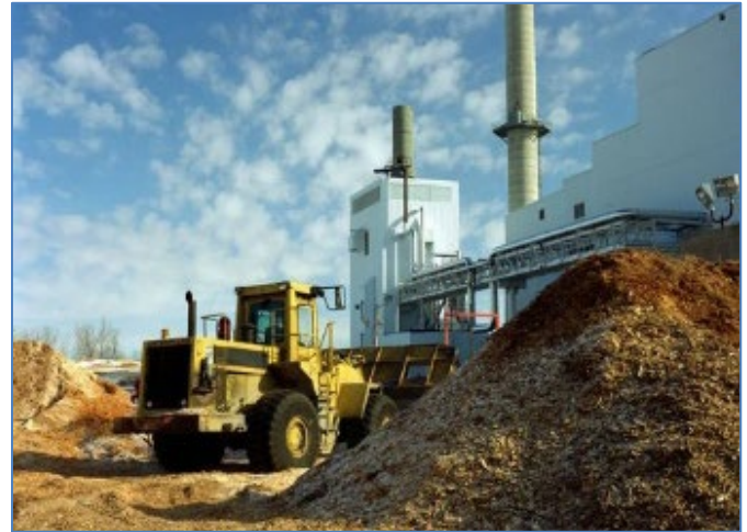
The McNeil Station biopower facility in Burlington, VT
