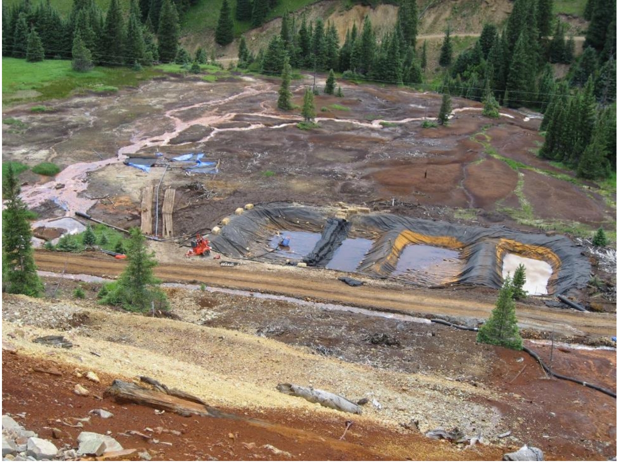
Pond lined with geo-textile fabric and filter bag system set up to west
