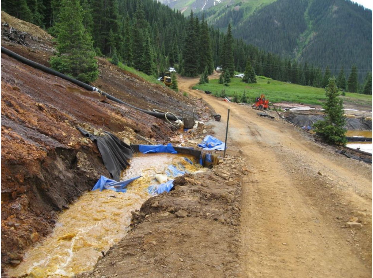
Mine water redirected to the settling pond during operations underground and treatment
