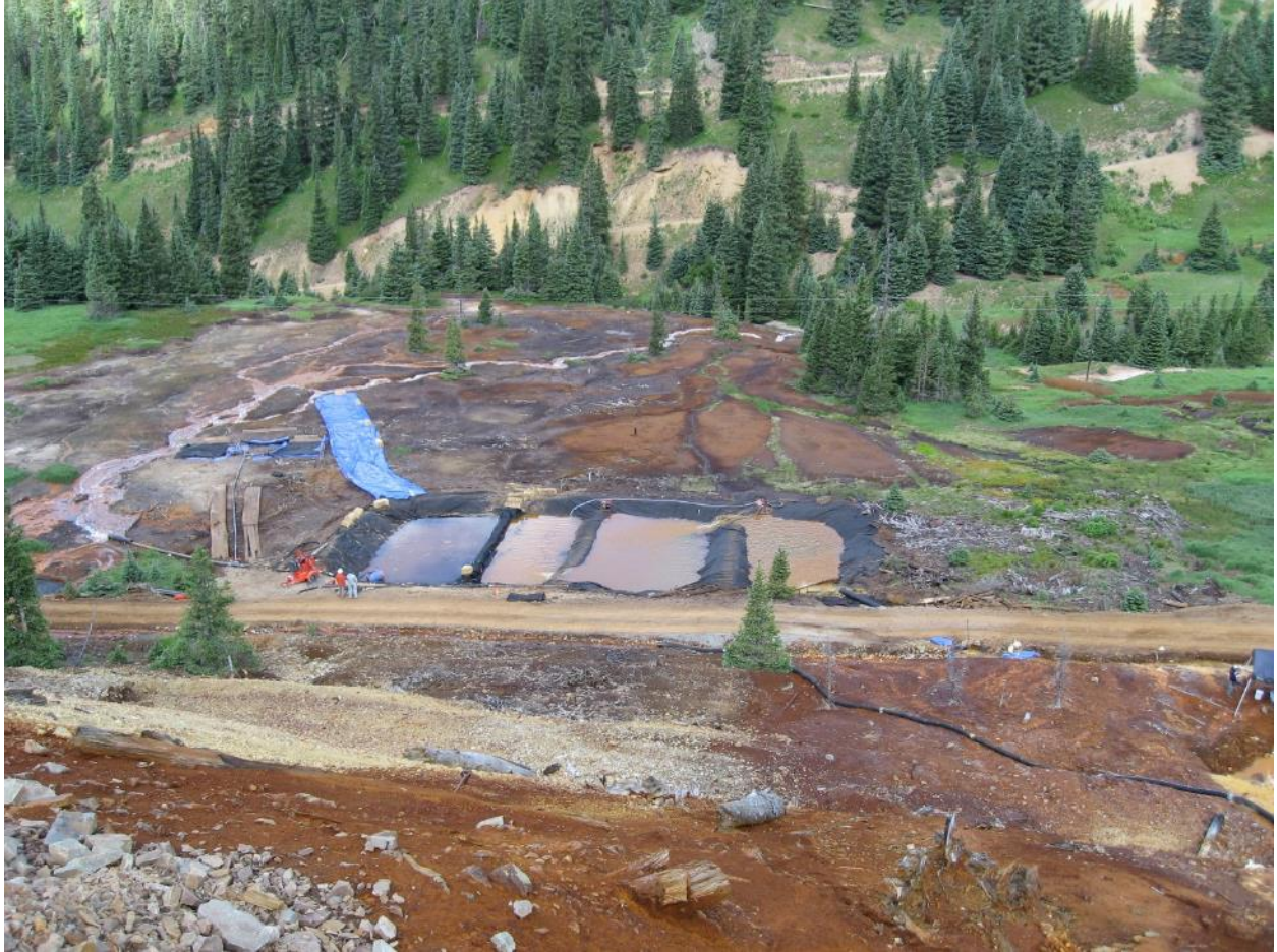
Discharge from pond after settling without filtering – lower turbidity than pre-work
