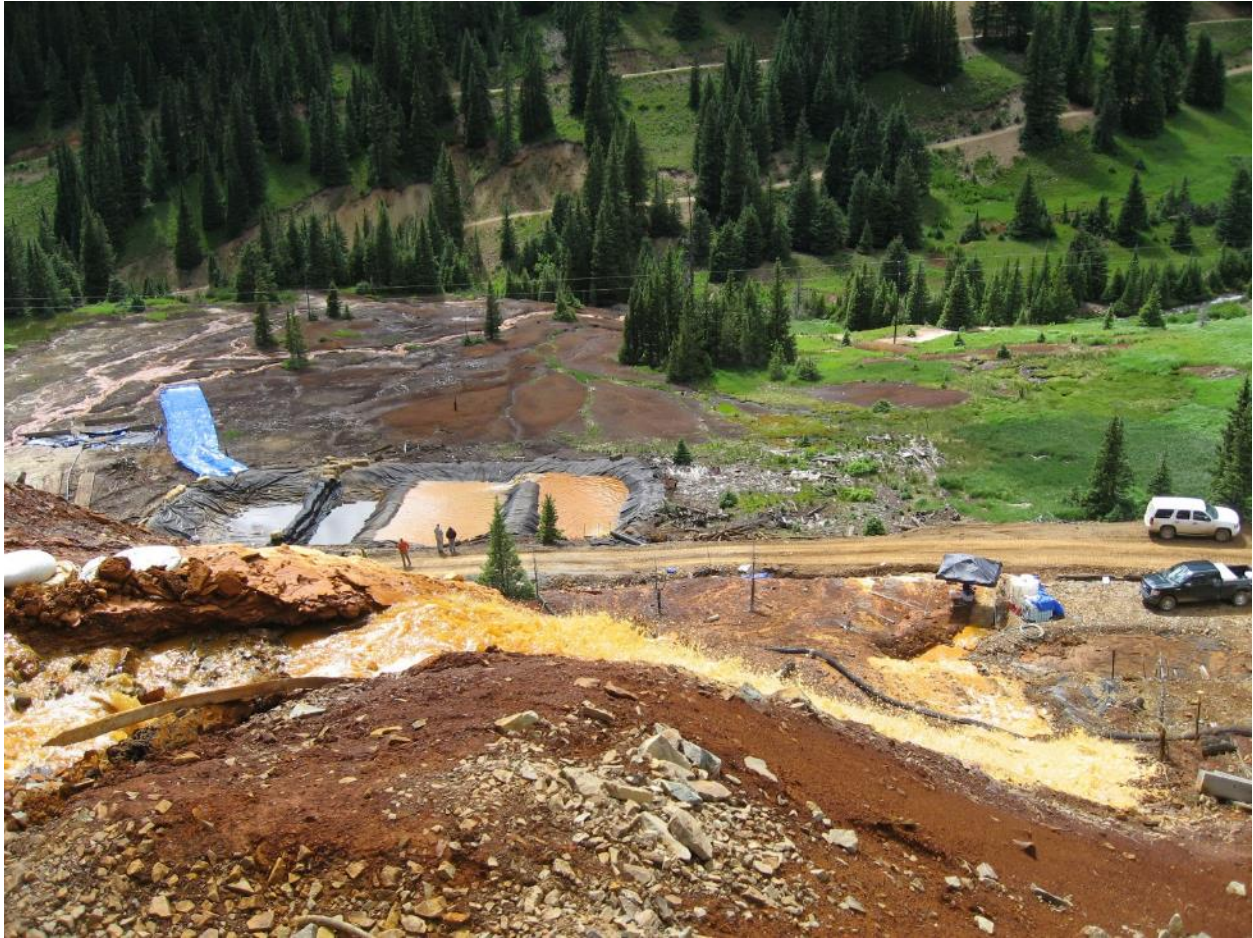
Retention/settling pond below waste dump – receiving mine water during underground operations July 21, 2015
