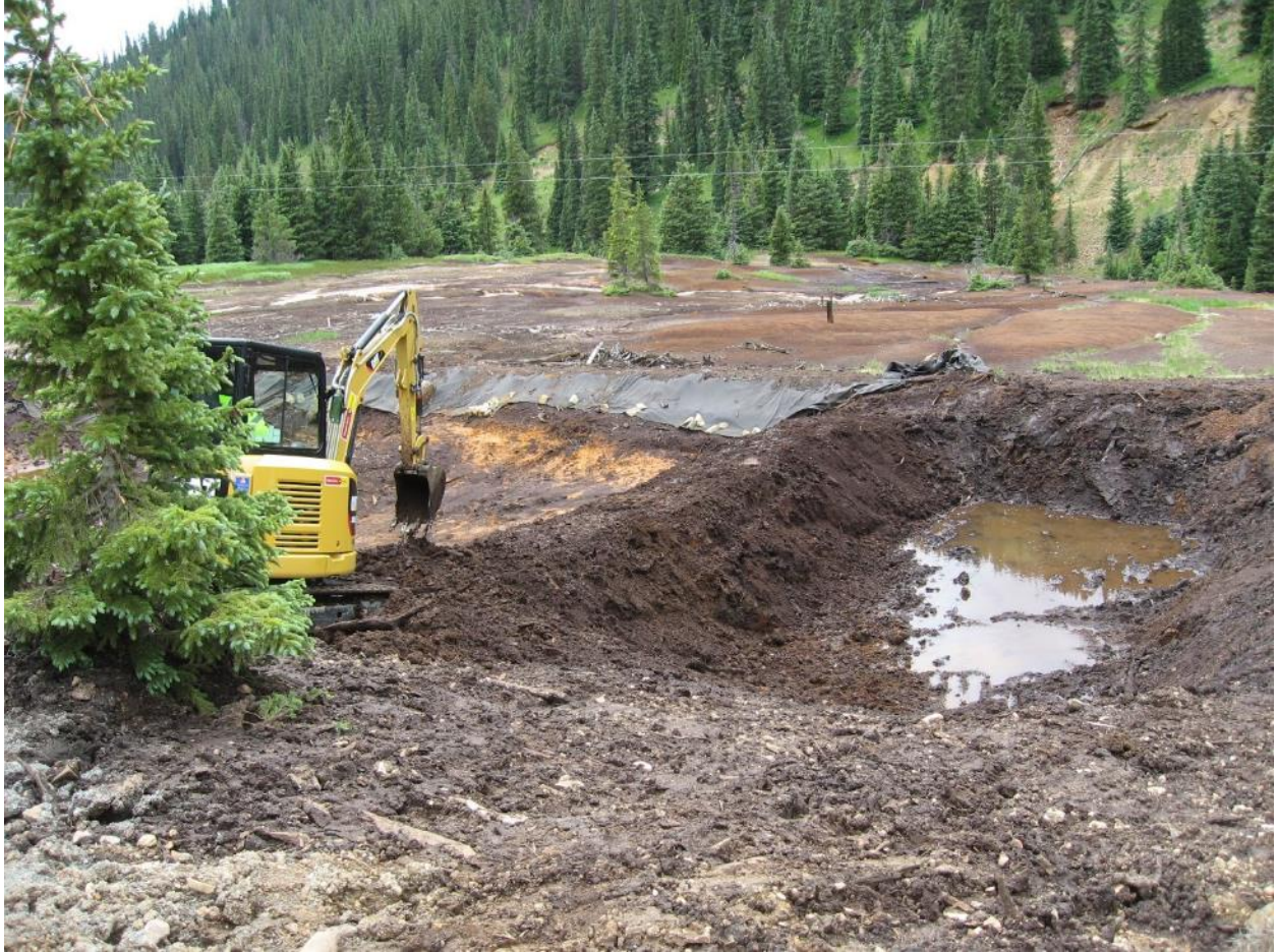
Pond preparation – expanded first cell and raising berms for increased storage
