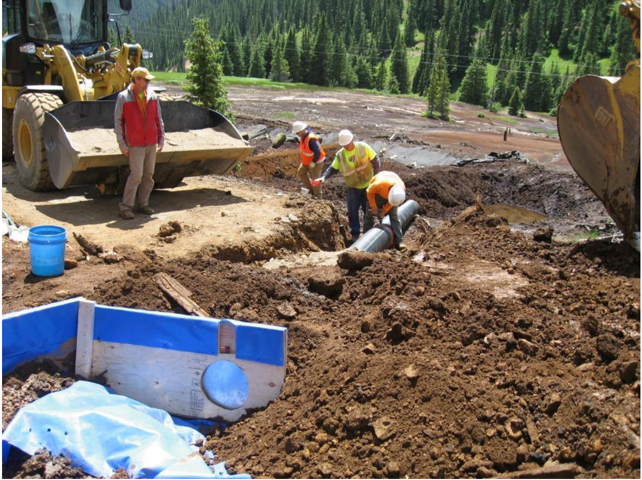
Headgates and pipe to pond
