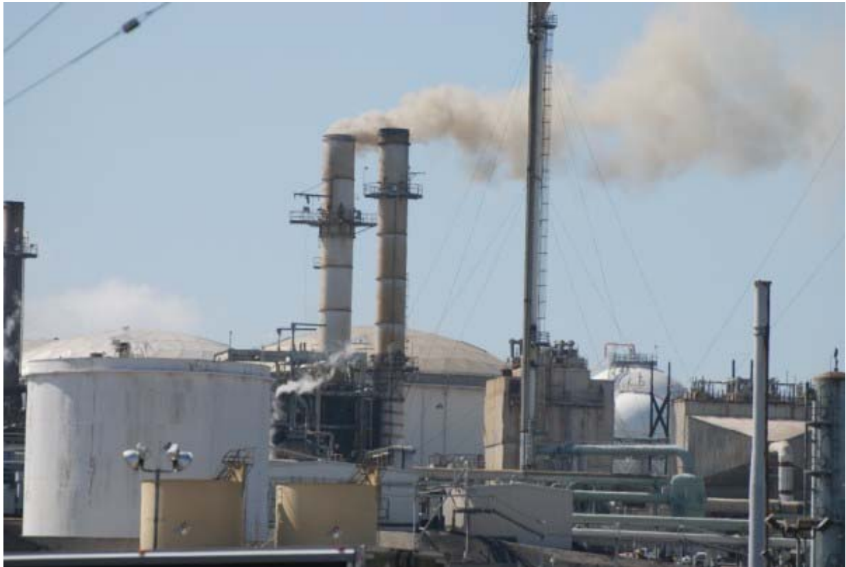
ConocoPhillips Wilmington Refinery October 5, 2007
