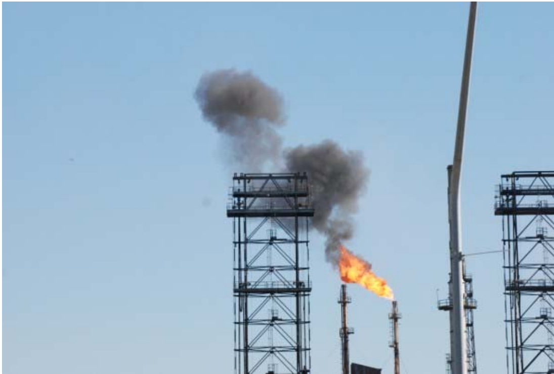
ConocoPhillips Wilmington Refinery February 5, 2008
