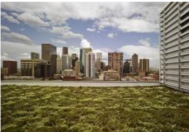
The EPA Region 8 building's green roof in Denver, Colorado, is an example of sustainable building practices used by the agency. The roof helps to regulate building temperature, reduce stormwater runoff and absorb carbon dioxide. (Source: EPA website)
