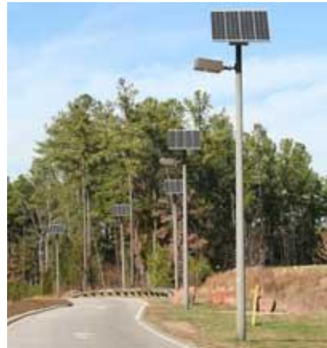
Solar lighting lines the roadways at the EPA's Research Triangle Park facility in North Carolina. According to the EPA, this is the longest stretch of solar-luminated roadway in the United States. Solar lighting is part of the agency's green power efforts. (Source: EPA website)
