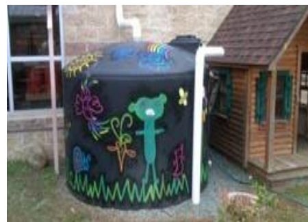
Water cistern used to collect and store rainwater for landscaping at childcare center at the EPA's Research Triangle Park facility in North Carolina. (Source: EPA website)
