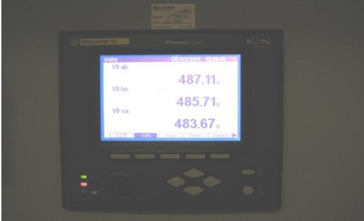
Advanced electric meter and boiler at the EPA's laboratory in Manchester, Washington. The EPA is required to install advanced metering equipment to capture energy consumption at its facilities to the maximum extent practicable. The EPA also initiated a project at its Manchester lab to retrofit fuel oil-fired boilers with natural gas to reduce GHG emissions and save on fuel costs. (EPA photos)
