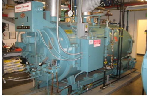
Advanced electric meter and boiler at the EPA's laboratory in Manchester, Washington. The EPA is required to install advanced metering equipment to capture energy consumption at its facilities to the maximum extent practicable. The EPA also initiated a project at its Manchester lab to retrofit fuel oil-fired boilers with natural gas to reduce GHG emissions and save on fuel costs. (EPA photos)
