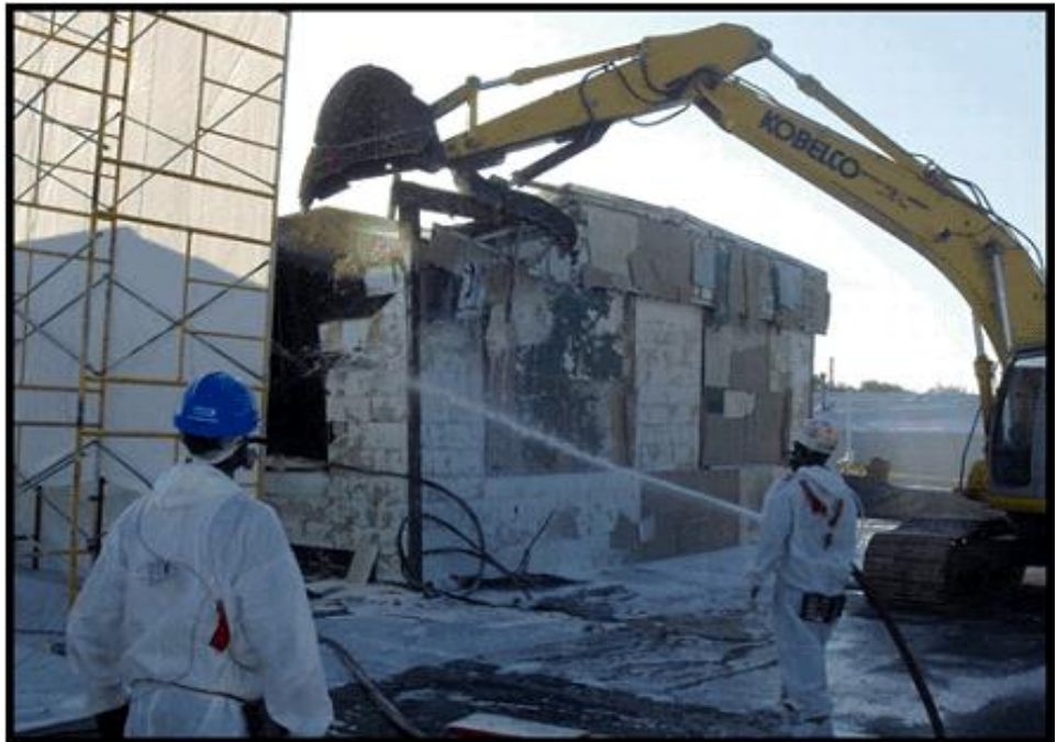
Demolition equipment prepares to break RACM during an AACM experiment. (EPA photo)
