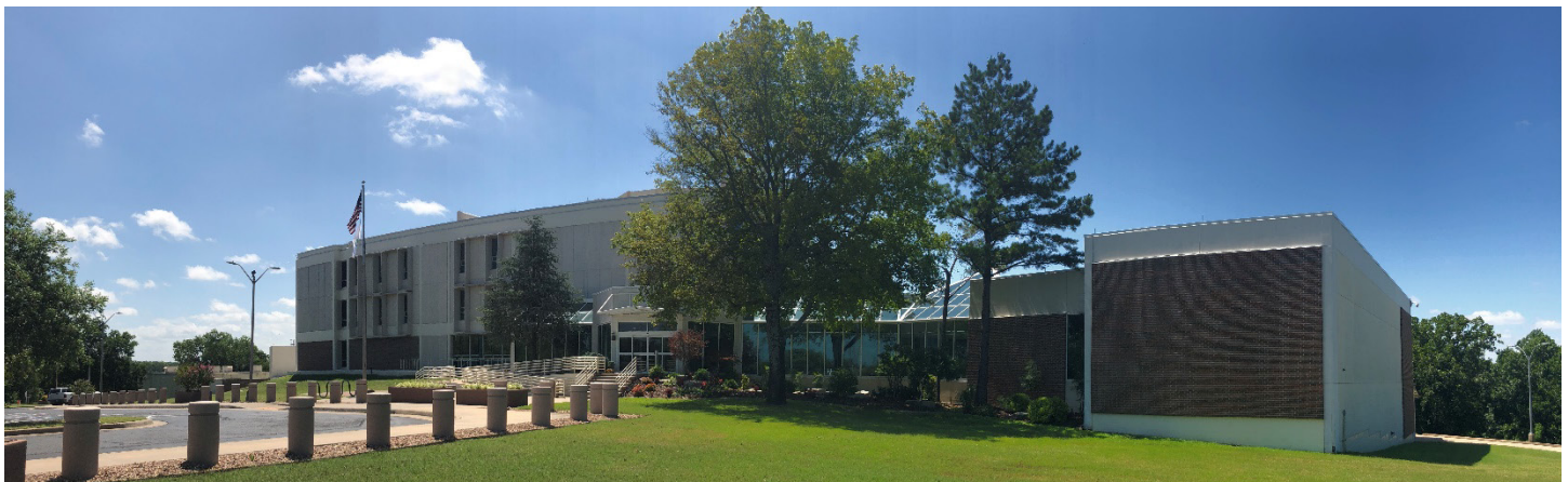
Figure 1. View of the Robert S. Kerr Environmental Research Center main building and library conference center (LCC).
