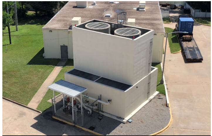
Figure 5: A 450-ton cooling tower provides space cooling for Ada's main laboratory and LCC.
