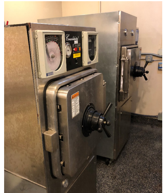
Figure 6: Two steam sterilizers at the ERC have on-board steam generation and only apply tempering water when in operation.
