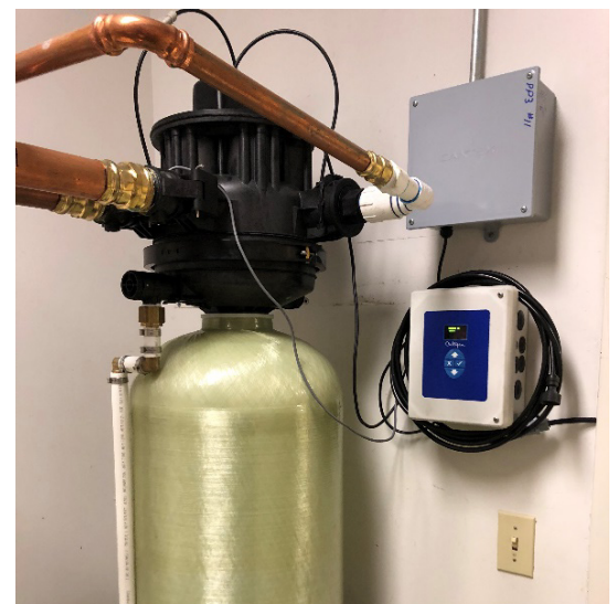
Figure 7: Ada installed a new water softener system for the LCC in November 2017 to replace an inefficient and malfunctioning unit.
