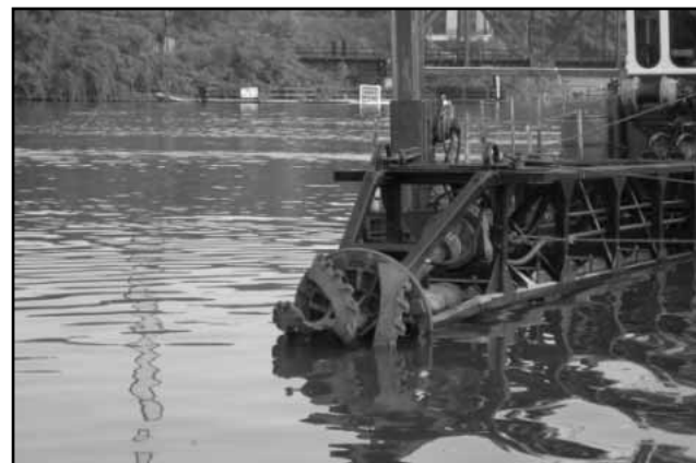
The hydraulic dredge used in the Ashtabula River to pump the contaminated sediment via pipeline to a disposal facility 2.5 miles from the river.
