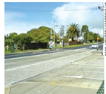
This monitoring site in Auckland, New Zealand, tested the effectiveness of permeable pavement on slopes.
