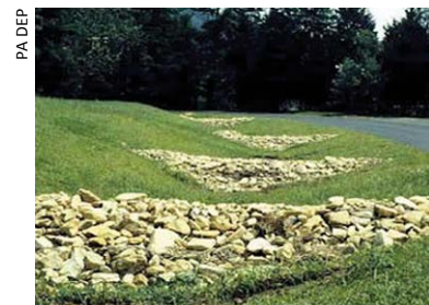
The rock check dams placed along this sloped, grassy swale help slow stormwater flow.
