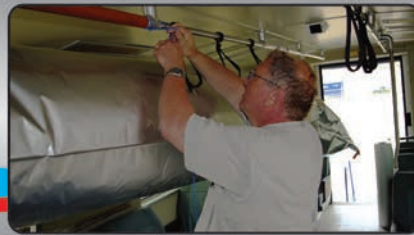
11 Installing Mylar displacement bladder so less methyl bromide is required during fumigation;
