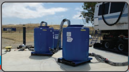
4 Carbon scrubbers built and ready to use;
