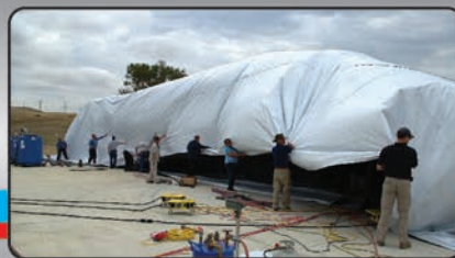
11 Installing Mylar displacement bladder so less methyl bromide is required during fumigation;
