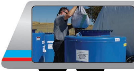
1 Setting up the carbon scrubber with coconut-based activated carbon;
