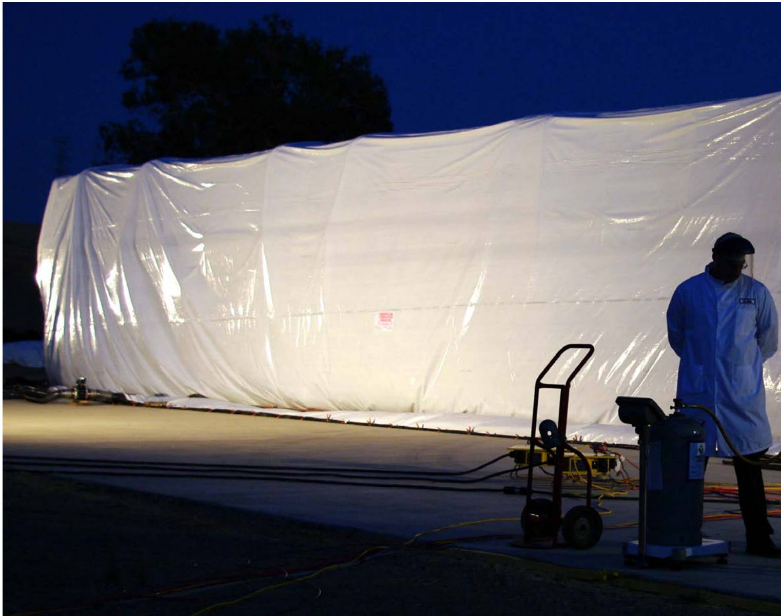
Shooting methyl bromide into a contained rail car at night.
