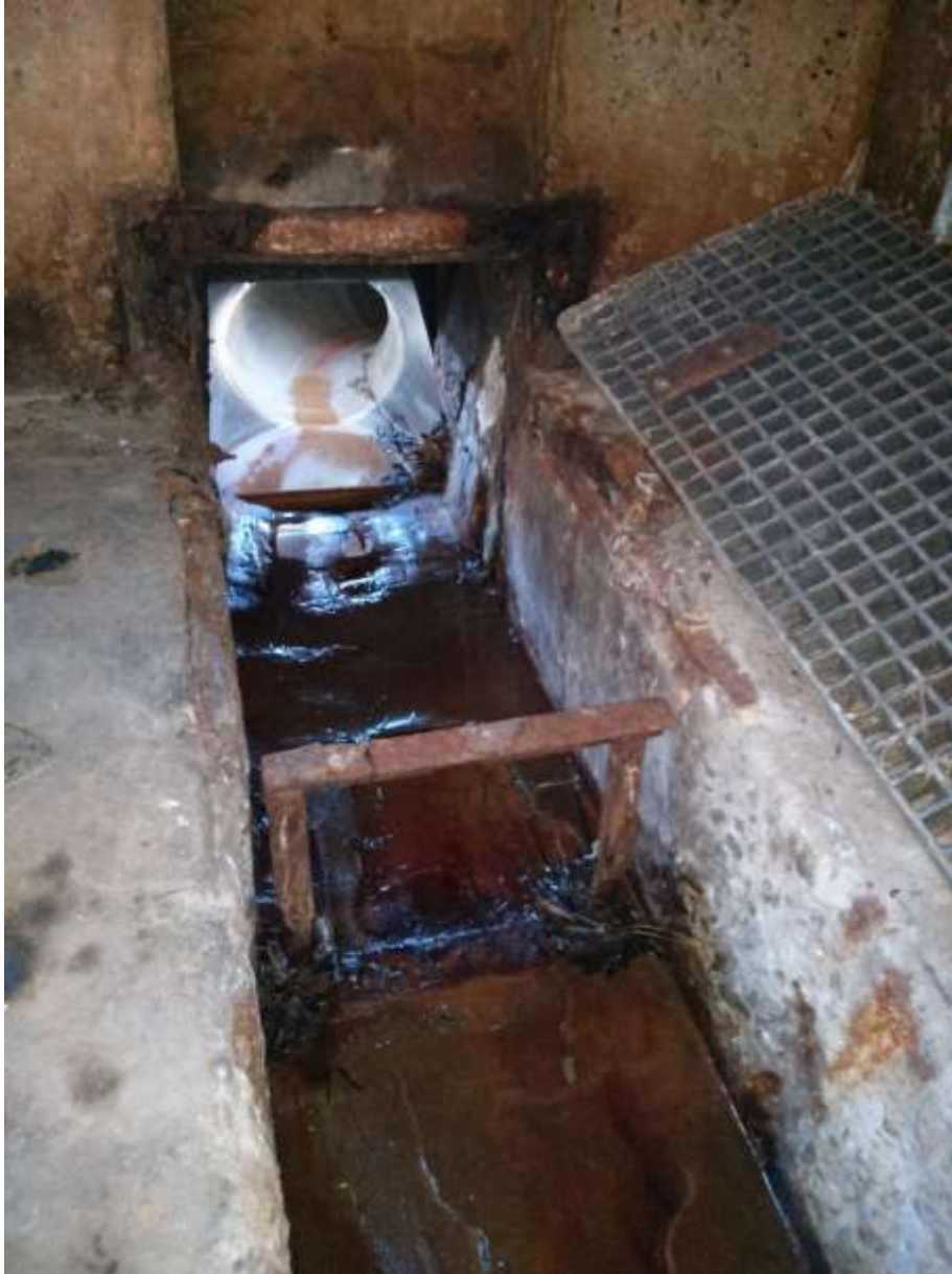
Figure 9-3: Unit 4 Fish Return Trough
