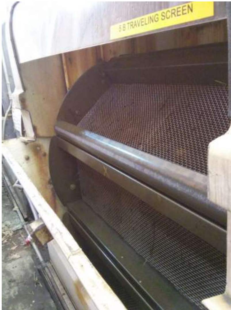
Figure 9-1: Schiller Station's Unit 5 Intake Screen
