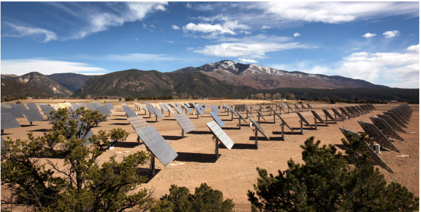
The Molycorp facility, a 21-acre concentrated photovoltaic solar system situated on a former mine site in Questa, New Mexico, has been fully operational since February 2011.
