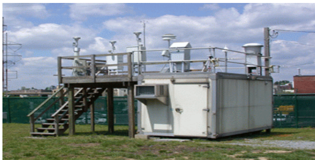
Ambient air monitoring station in Wilmington, Delaware (Delaware Department of Natural Resources and Environmental Control photo)
