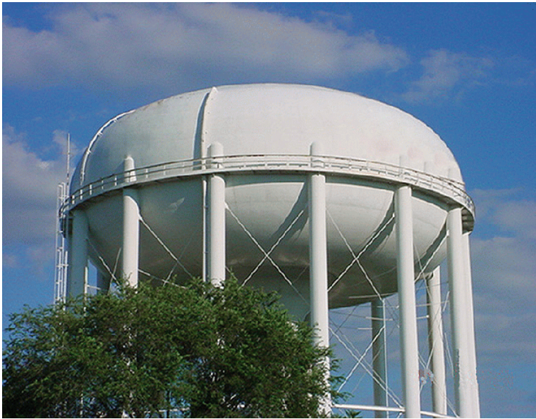
A water tower in New Jersey (EPA OIG photo)
