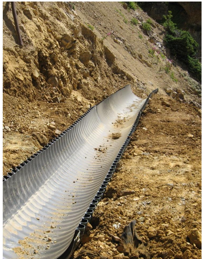
2008 – Installation of permanent portal discharge diversion structure
