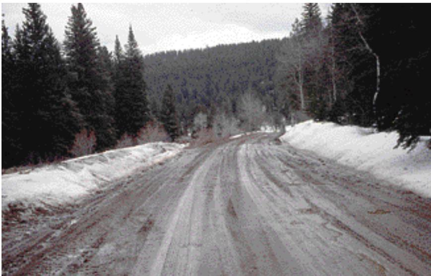
Remarkable difference in these two roads that carry similar volumes of traffic. They are located in the same region of the country and the photos were taken on the same day. The major difference is drainage. The upper photo shows a well-drained road while the lower photo shows a poorly maintained ditch that resulted in a poor performance.
