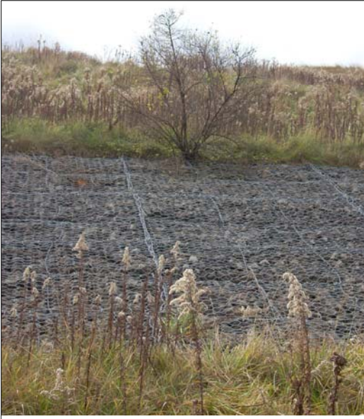
View of rip-rap at the capped and stabilized slide mound, used to keep the mound in place. (EPA OIG photo)
