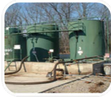
Deep well injection
