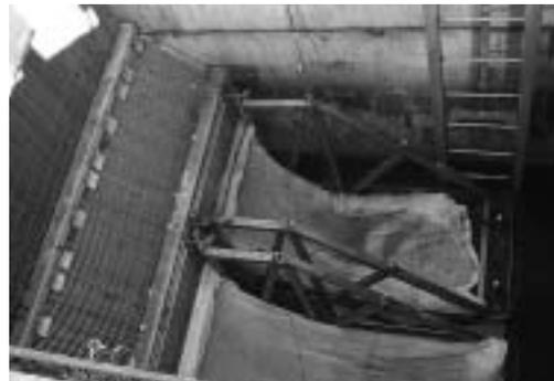
Photo: Solids and floatables controls, such as the nets pictured here, are installed at all North Bergen CSOs. *Courtesy of NJDEP*
