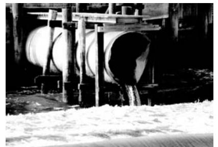
Typical CSO outfall discharge following a storm.
