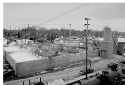
Since the passage of the Clean Water Act in 1972, all levels of government have made substantial investments in the nation’s wastewater infrastructure.
