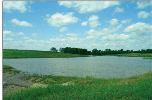
Figure 2. Example of a sediment pond constructed along a tributary stream in an agricultural watershed. The pond is designed to remove suspended and soluble nonpoint source pollutants.
