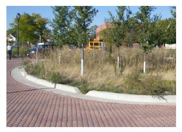
Above: A rain garden in a roundabout designed to capture and infiltrate stormwater in Milwaukee, WI. Left: Rendering of a curb bumpout along a residential street. Below: Cut-away of a curb bumpout with permeable pavers on sidewalk.
