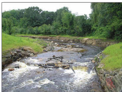
Figure 2. Same location as Figure 1, showing Black Brook in June 2009 after the dam was removed and natural gas line relocated.
