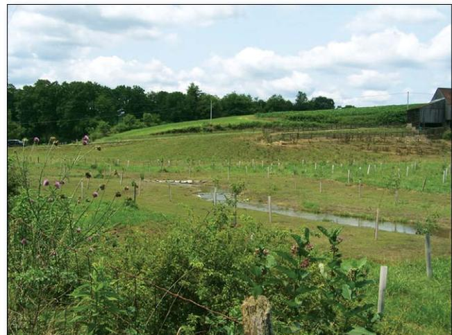
Figure 1. Watershed partners restored this section of Pennsylvania's Pierceville Run by grading streambanks, planting a riparian forest buffer and installing fences to prevent cattle access.
