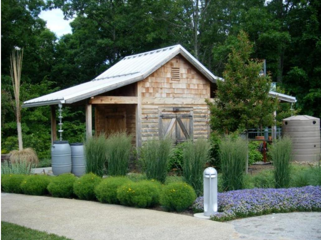
Figure 3-7. Rain barrels adequately sized for contributing roof area.
