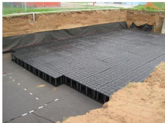
Figure 3-8. Subsurface infiltration gallery.
