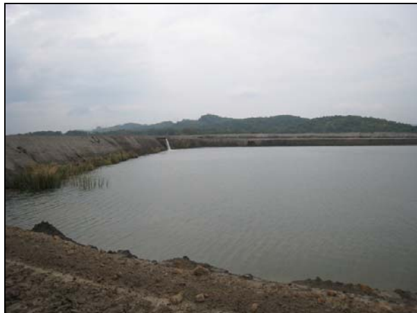
Surface impoundments accumulate high concentrations of toxic pollutants from fly ash transport water, bottom ash transport water, and FGD wastewater.
