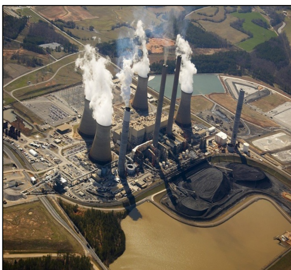
Georgia Power Company's Plant Bowen
