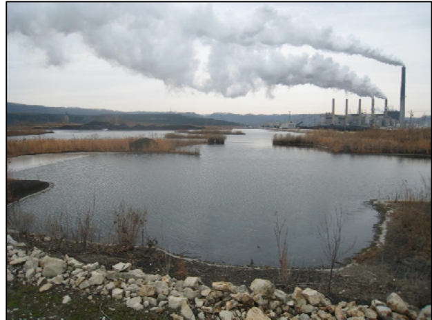
Surface impoundments and constructed wetlands can act as attractive nuisances by attracting wildlife and exposing them to elevated pollutant levels.
