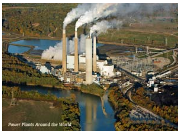
IPL's Petersburg Generating Station
