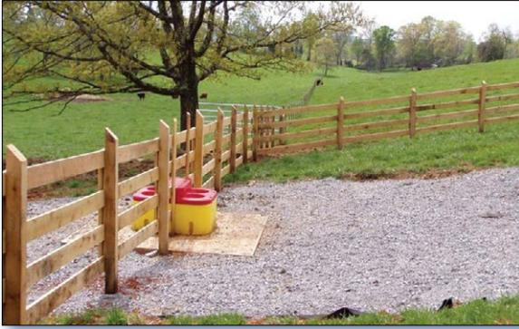
Figure 2. Landowners installed BMPs like this watering system for livestock, which includes exclusion fencing and heavy-use area protection.
