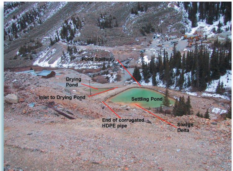
The mine drainage treatment system mixes kiln dust with acidic runoff to increase the pH of the drainage water. Once a pH of between 9.5 and 10 is achieved, metals are precipitated out in a settling pond and the clean water is returned to the creek.
