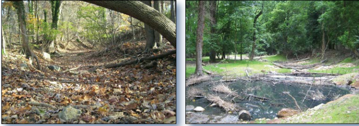
Figure 2. The Broad Branch tributary was previously confined to a pipe buried under the original stream valley (left). The daylighting project restored the stream to the surface (right).
