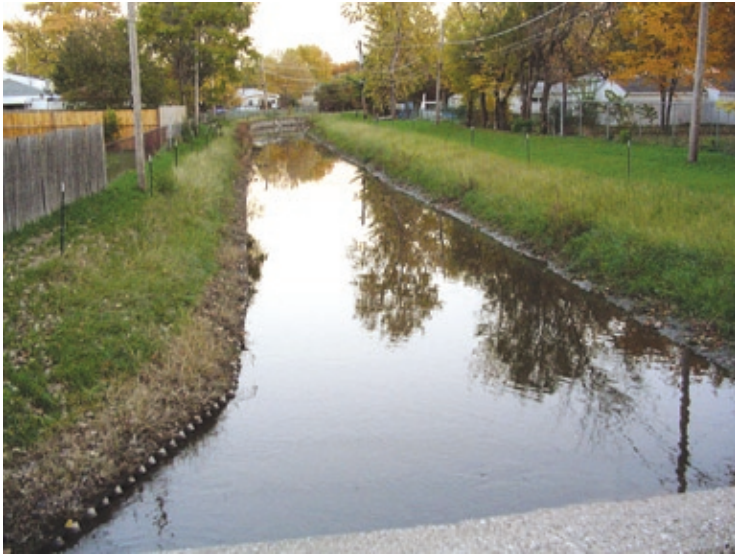
Figure 3. Streambank stabilization techniques used on this portion of the creek include vegetated banks with an A-Jacks toe on the left bank and a Stabilator toe on the right bank.
