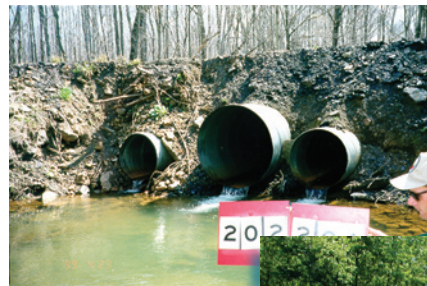
Photos of the culvert/fish blockage taken before and after the Neff Run Phase I project show significant improvement. (Photographs courtesy of Maryland DNR's Watershed Services Center)
