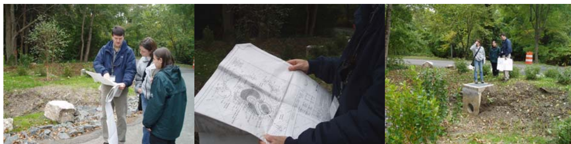
Figure 2. While comparing an existing STP to the original plans, the field team realized the trash rack was never installed.
