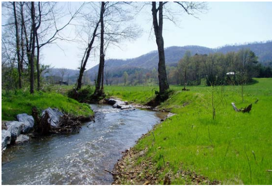
After: The rebuilt channel was designed with a more stable pattern, modeled after a similar, relatively undisturbed stream.
