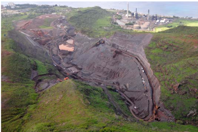
Waste Management of Hawaii's Waimanalo Gulch Landfill after the massive rain events in December 2010—January 2011. Waste Management never installed the stormwater diversions required by their permit which is what caused the flooding and pollutants to be discharged.
