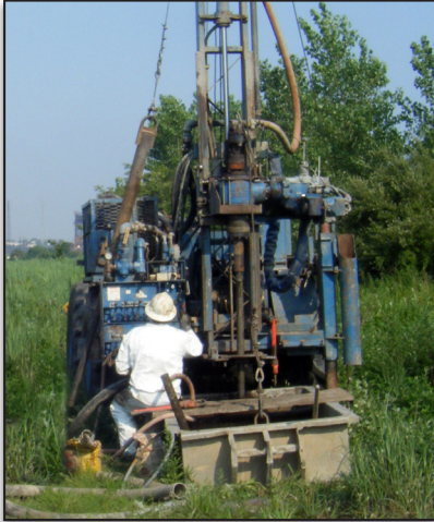
Site Investigation: Drilling
