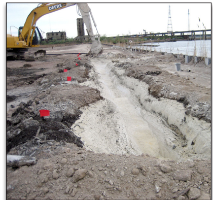
Slurry Wall Installation
