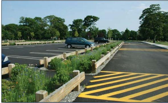
Figure 2. Project partners installed vegetated bioinfiltration swales in this parking lot near the beach.
