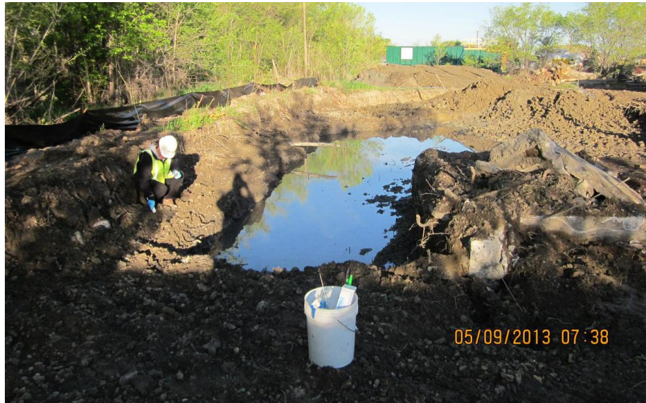
Confirmation soil sampling around outside of removal area at Murray Laundry site. (EPA website)
