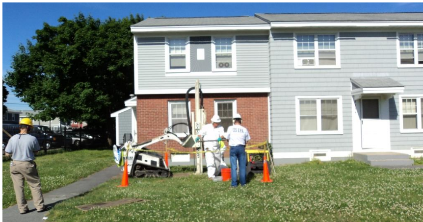
Removal action work being conducted at Parker Street Waste Site. (EPA website)
