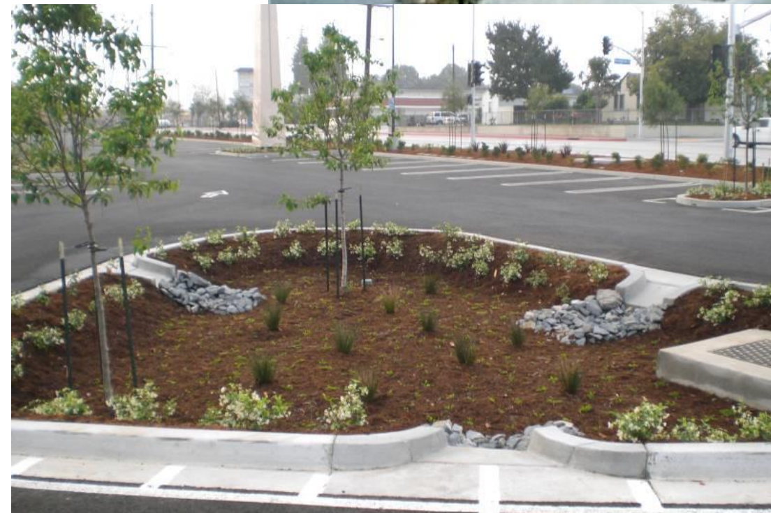
Bioretention Cell in El Monte, CA. Photo courtesy of Bill DePoto.
