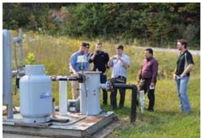
Site tour participants visit the flare station at EnergyXchange in North Carolina
