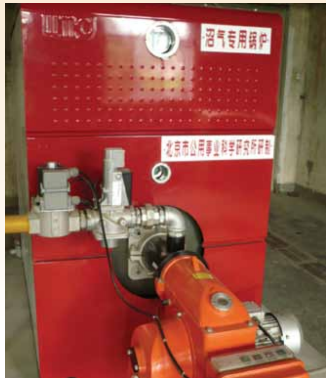
LFG-fired boiler in operation at Gaoantun Landfill in China
