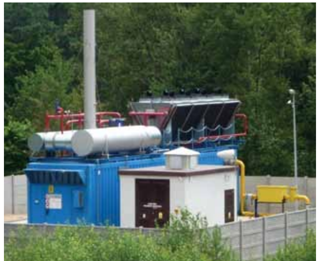
CHP unit at abandoned Zory Coal Mine in Poland
