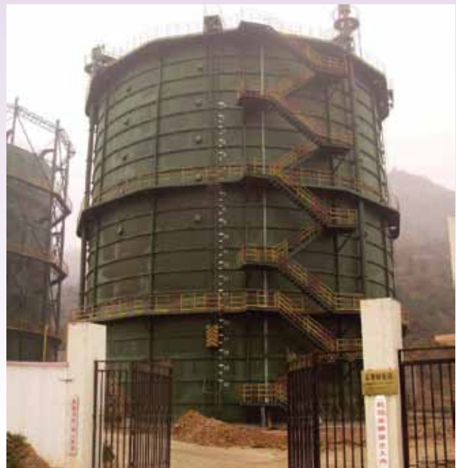
Expanding mine gas storage silo in Southern Shanxi, China
