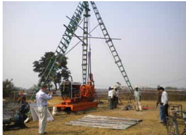
Drilling cores in the Damodar Valley, India
