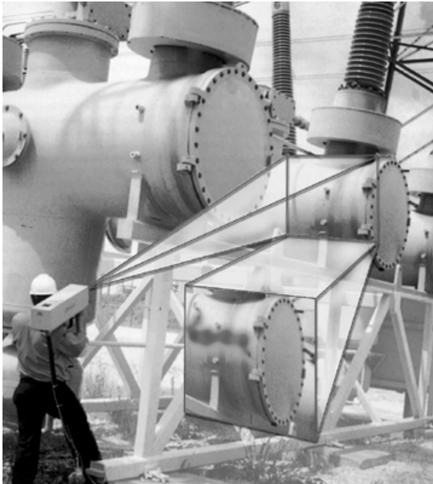
FIGURE 2. Leak Location Using a GasVue System
