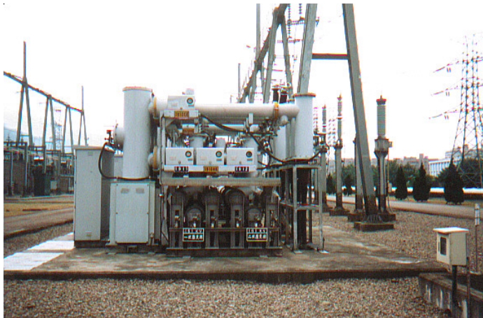
GIS(Gas Insulation Switchgear)
