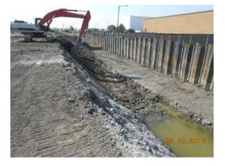
Photo 2: Excavation along ERS at Area 5S
