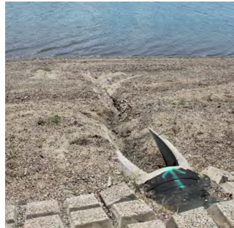
Figure 10: Pierre's stormwater system draining directly into the Missouri River.
