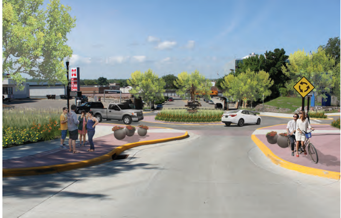
Figure 22: Design concept for the intersection of South Pierre Street and Pleasant Drive. The major design option at this site is a roundabout added to the intersection of South Pierre Street and Pleasant Drive. A roundabout could benefit this area by simplifying traffic patterns, slowing the average traffic speed, and creating safer and shorter distances for pedestrians to cross the street. Stormwater planters, street trees, and aboveground planters could calm traffic while adding visual appeal to the intersection.
