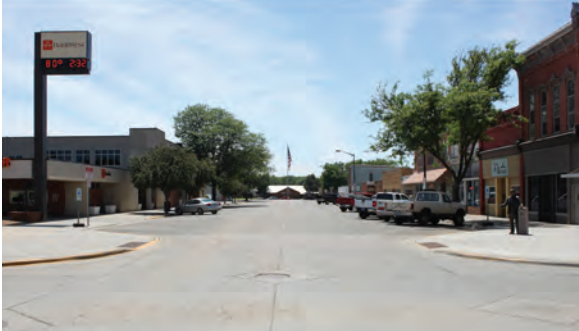
Figure 26: Current condition of the block-long segment of South Pierre Street between Dakota Avenue and Missouri Avenue.
