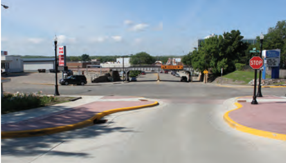
Figure 21: Current condition of the intersection of South Pierre Street and Pleasant Drive.
