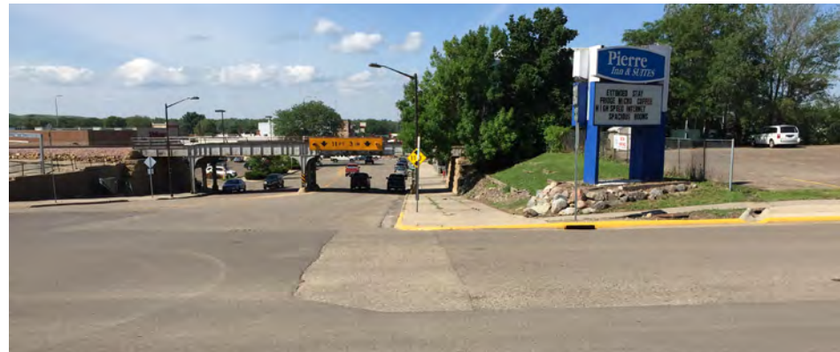
Figure 7: View to the south from the corner of Pleasant Drive and South Pierre Street where South Pierre Street goes under the tracks.
