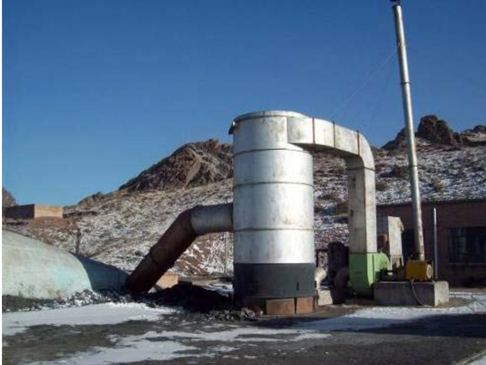
Figure 1.9: Example of Current Ventilation Drift Heating Arrangements
