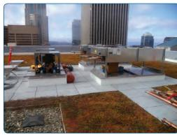
Above: The new cooling system takes air from the outside and filters it into the server/network room at much lower cost than the previous air conditioning units.
