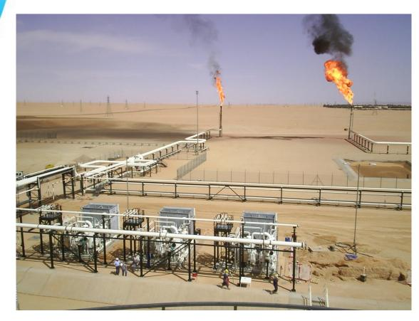
Picture of the flares at NC-115 after the VRU's were installed. Units capturing 4 MMscfd (Four million standard cubic feet per day) of previously flared or vented natural gas streams.
