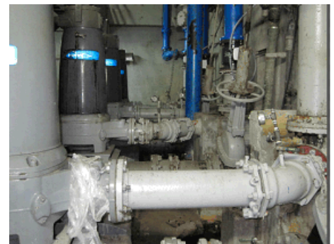
Newly installed pipes and valves at Fujita Pump Station. (EPA OIG photo)
