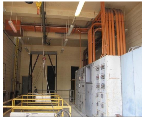
Control Bay at Route 16 Pump Station. (EPA OIG photo)
