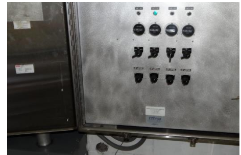
Control panel at Fujita Pump Station. (EPA OIG photo)
