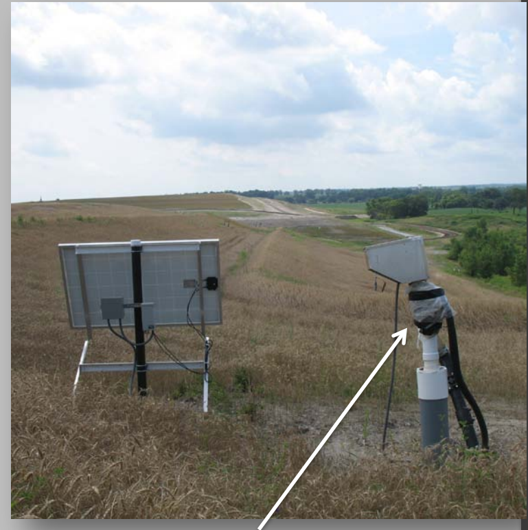
Site installed simple insulation below driver
