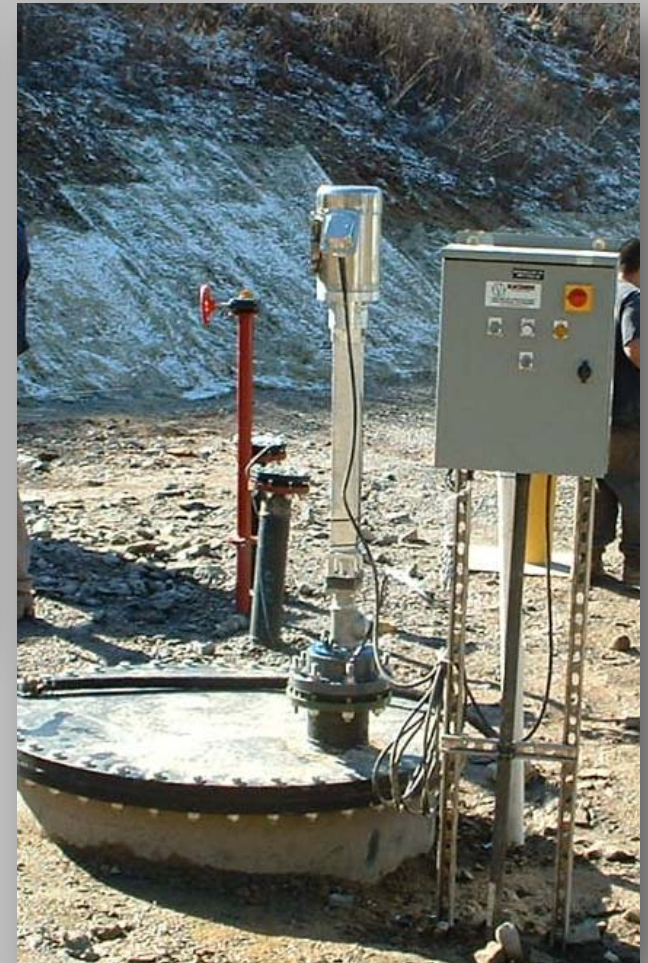
Anchor Electric, with Controller
